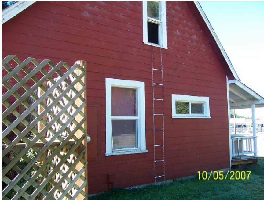
Outside of the unit with the ladder ready for evacuation
